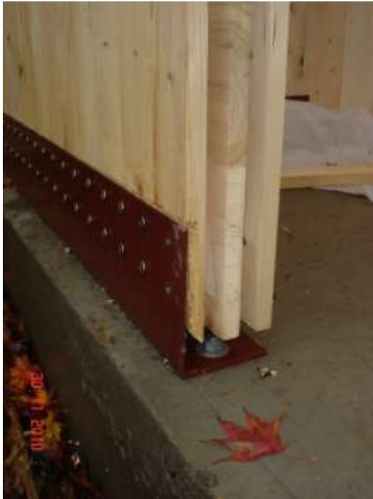
Double internal spline
