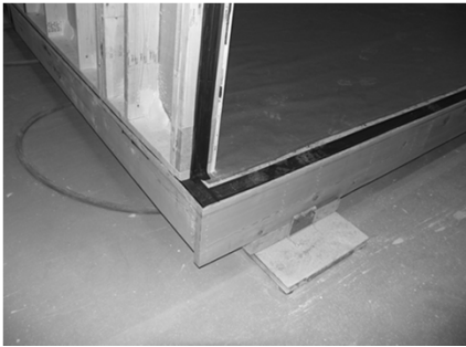
EPDM gasket at floor and wall intersections
