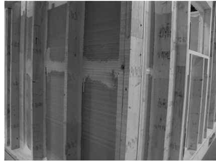
Foam sprayed on sheetrock joints at tub to complete air-seal
