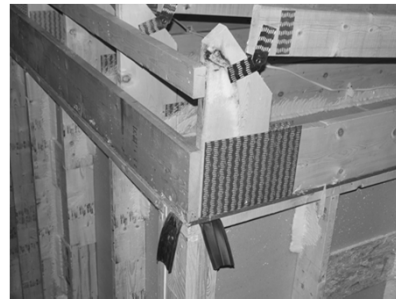
20" raised Heel folding truss w/ EPDM gasket between walls and ceiling
