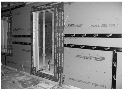
Air sealing of wall sheathing
