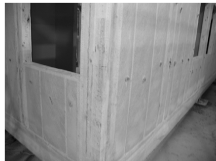
Installed dense pack cellulose
