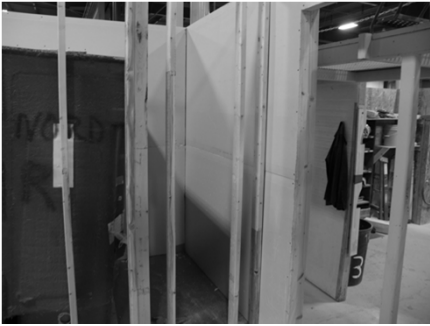
Full sheetrock air-seal behind tub
