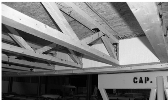
4" Foam blocking on outside perimeter of floors – open web joists – urethane adhesive on floors
