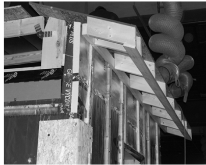
Eave framing on shed roof
