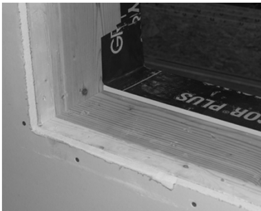
13 3/8" window buck clapboard drainage under window
