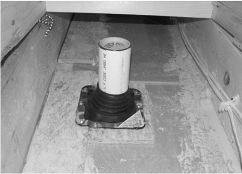
Air seal around plumbing vents
